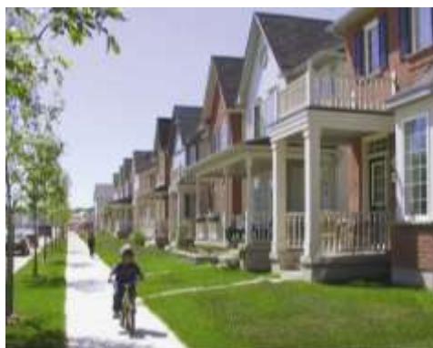
The City is expanding towards its outer edge through sensitive suburban development
